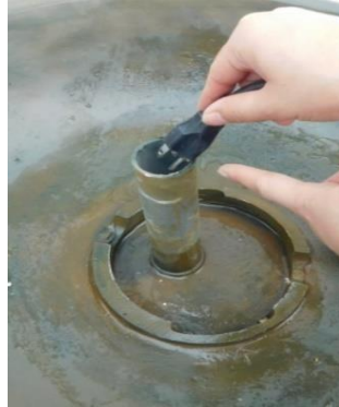
Pass the power cord from the pump down the cord pipe and through the pedestal.
