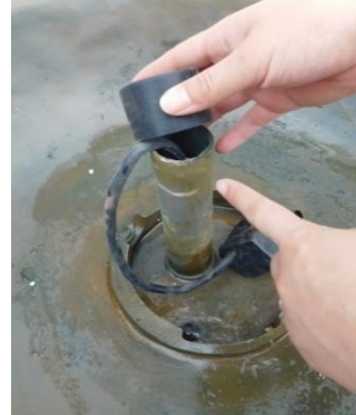
Install the cord pipe cover over the cord pipe as shown above.
