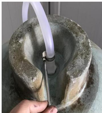
Secure the tubing to the bowl with the fastener as shown.
