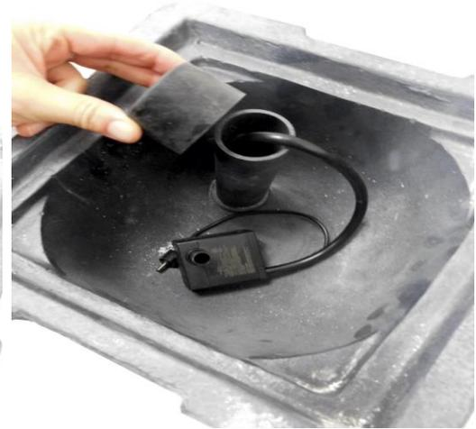
Install the cord pipe cover over the cord pipe to prevent any chance for water-loss.
