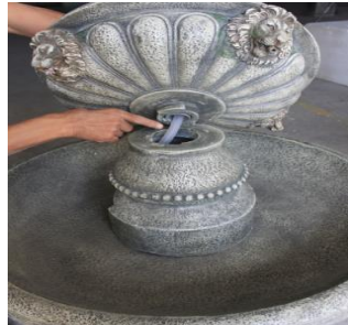
Feed the tubing up the pump housing and pass it through the centre of the middle bowl.
