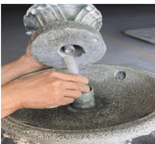
Connect the tubing to the top.
