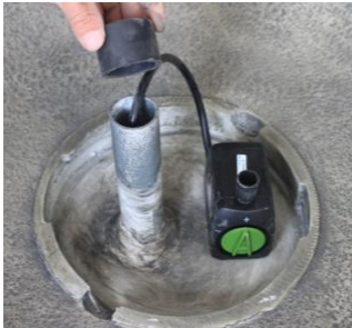
Install the cord pipe cover by aligning the cord then fitting it over the pipe and cord.
