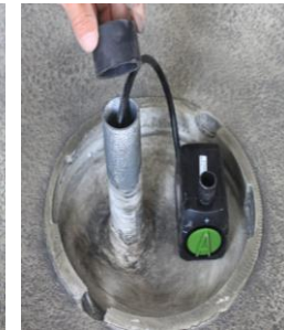
Install the cord pipe cover by aligning the cord then fitting it over the pipe and cord.
