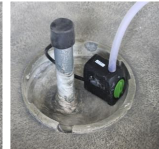
The pump should sit flat inside the bowl as shown. Attach the included tubing to the pump.
