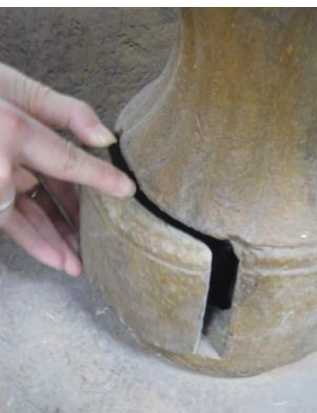
Install the pump access door.
