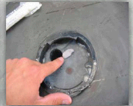
Apply putty to the leaking area.
