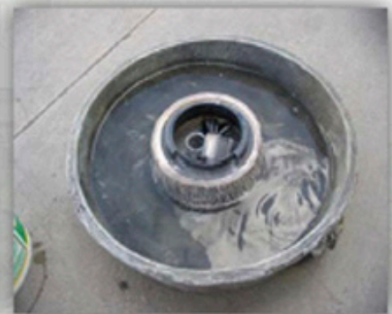
Allow bowl to sit. Look for leak.
