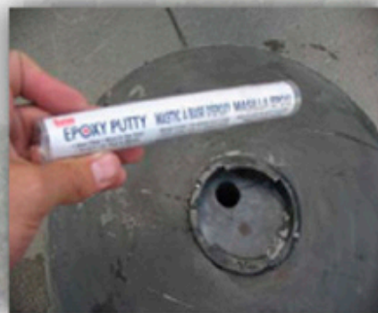
For this repair, Oatey Brand Epoxy was used.
