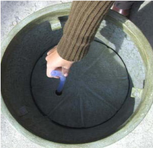
Proper plate and tube placement
