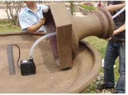
Carefully place the largest riser in the bowl at an angle as shown. Attach the tubing to the pump and pass it through the riser.
