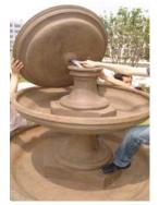
Carefully rest the smallest bowl on its edge. Pass the tubing through the bowl as shown above.
