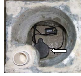
Place the cord pipe cover over the cord pipe as shown above.
