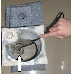
Feed the cord down the cord pipe and align with the groove at the base.
