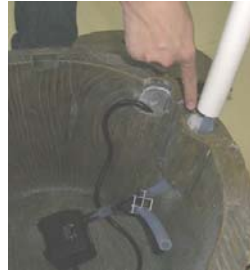
Slide the "slip fit" pipe into this same hole. Feed the tubing up through the hole.
