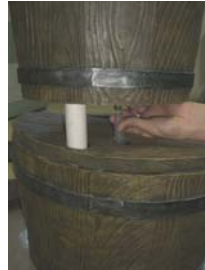
Set the bowl in place by sliding it down over the white pipe. Connect the tubing from the previous step to the outlet on the bottom of this bowl. Carefully set the bowl in place.
