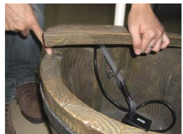
Set the large cover plate into place on top of the bowl by aligning the grooves.
