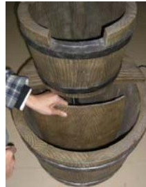
Install the pump access door.
