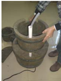
Set the bowl in place by sliding it down over the white pipe. Connect the tubing from the previous step to the outlet on the bottom of this bowl. Carefully set the bowl in place.
