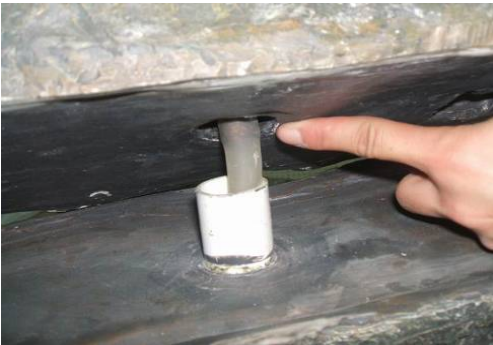
Slide the top piece of the fountain over the slip fit mechanism and into place.
