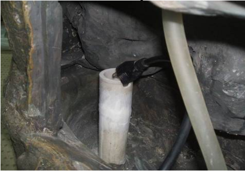
Run the pump cord down the cord pipe.
