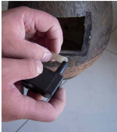
Locate the tubing from inside the fountain and connect it to the pump.
