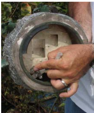
Note restrictor for fine tuning of flow
