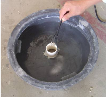
Feed the pump cord down through the cord pipe and align with groove at the base.
