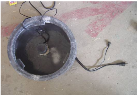
Install cord pipe cover.
