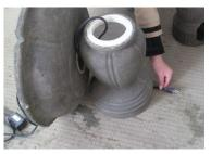
Pass the pump cord through the pedestal and align the cord with the groove at the base.
