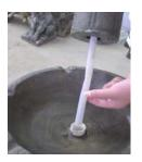
Feed the tubing from the top section down the pipe as shown above.
