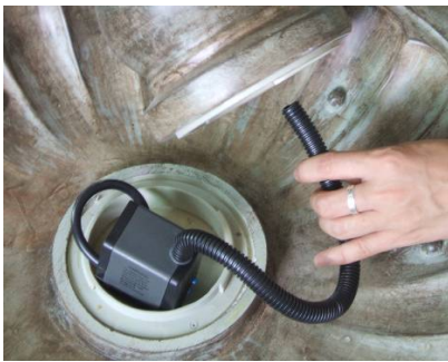
Connect tubing to pump. Run tubing up through the riser.
