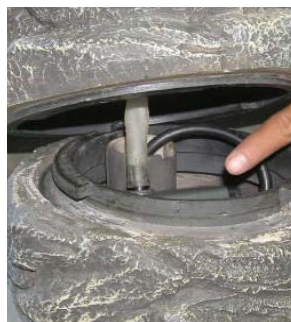
Place pump in housing be sure not to kink hose
