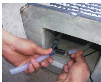
Connect the tubing from the light to the "Y" connector.
