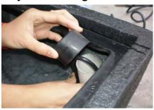
Install the cord pipe cover by fitting the rubber cap over the pipe.
