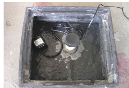
Install the cord pipe cover.
