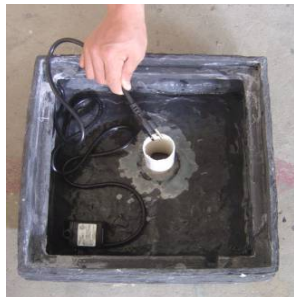
Feed the pump cord down through the cord pipe.
