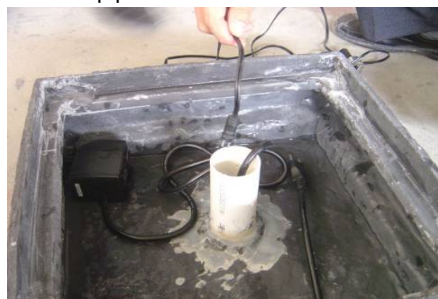
Feed the pump cord down through the cord pipe.
