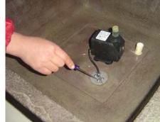
Once you have positioned the pump, ensure the cord seal is tight and secure.
