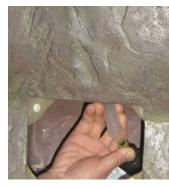
Connect the pump to the tubing from the top through the pump access opening. Be sure the pump is sitting flat and the tubing is not kinked.
