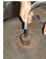
Feed the tubing and light cord from the top through the opening in the middle plate and down into the pump housing/riser.
