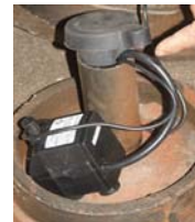
Pass any excess light cord down the cord pipe. Reach in through the pump door and install the cord pipe cover as shown.
