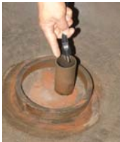
Feed the power cord from the pump down the cord pipe in the bowl.
