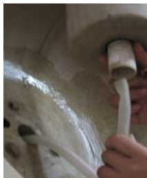
Run tubing through the final riser
