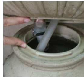
" Twist and lock" riser and bowl
