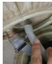
Install the " T" joint. Connect the short piece of tubing to the copper output. The long piece will go through the second bowl.
