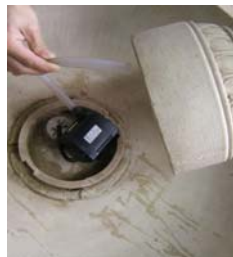
Connect tubing to the pump.
