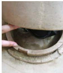
Install riser as shown
