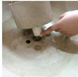
Slide the riser into place.
