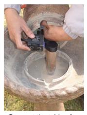
Connect the tubing from the top to the pump.
