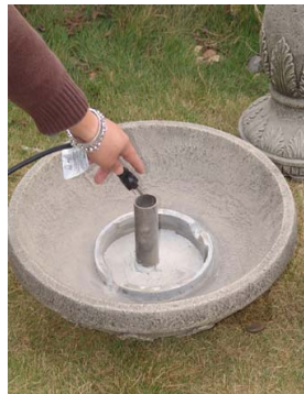
Pass the power cord down the cord pipe in the bowl.
