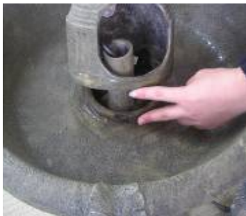
Twist and lock the riser to the bowl
