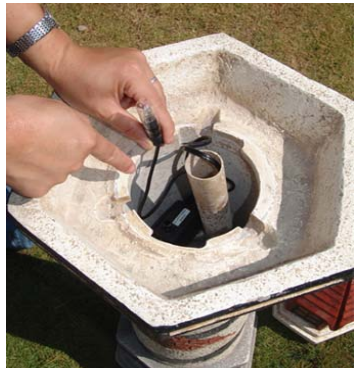
Place the pump and attached light inside the water reservoir.
