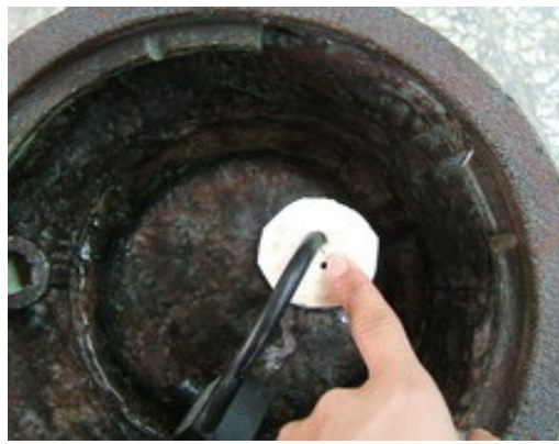
Install the pipe seal as shown.
