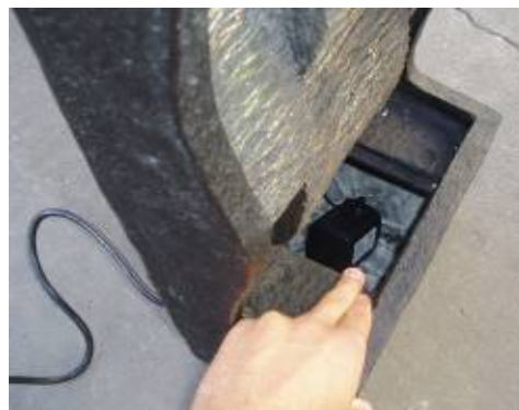
Set pump inside fountain and connect to tubing.
