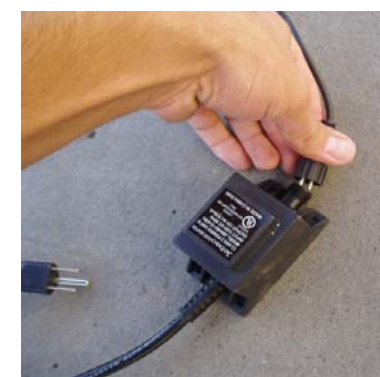
Connect the light cord to the transformer.
