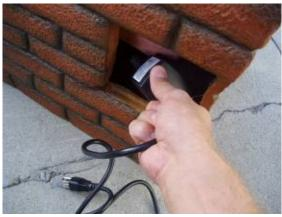
Insert the pump into the opening at the back of the fountain and connect to the tubing from the top.
