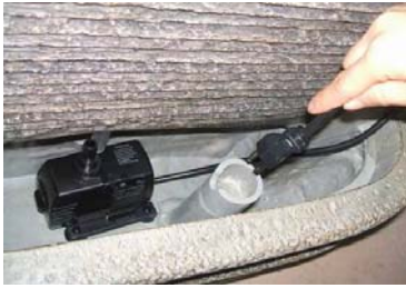
Pump cord through standpipe.
