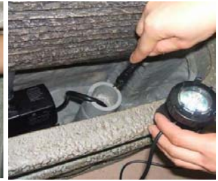
Light cord through standpipe.
