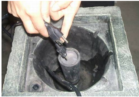
Pump and light cords through PVC pipe
