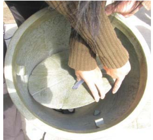
Rest baffle plate on notches, with tube directly above pump.
