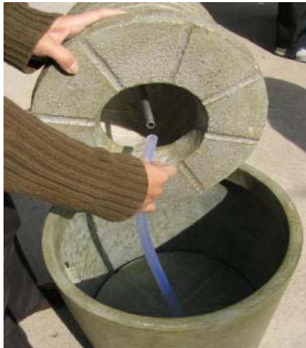
Attach tube to metal pipe
