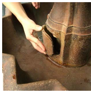
Install the pump access door.
