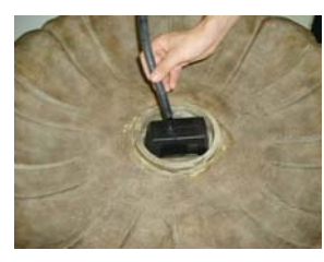
Connect supplied tubing to the pump as shown above.
