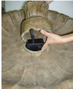
"Twist and lock" riser in place.
