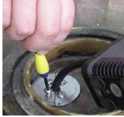
Pump comes pre-installed with cord seal. Check to see the cord seal is tight. Adjust pump to desired setting.
