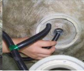
Install the " T" joint. Connect the short piece of tubing to the copper output. The long piece will go through the second bowl.
