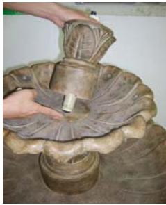
Run the tubing up to second riser. Slide the riser into place as snow
