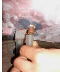
Feed the long tubing through the rear hole of the second bowl. Connect the other tube to the copper outlet.
