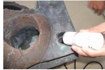
Insert the PVC pipe into place
