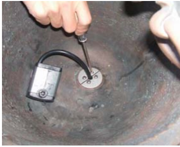
The pump and cord seal are pre-installed. Ensure the cord seal is tight.
