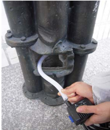
Locate the tubing from inside the fountain and connect it to the pump.
