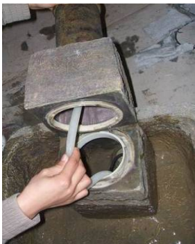
Run tubing through riser section.
