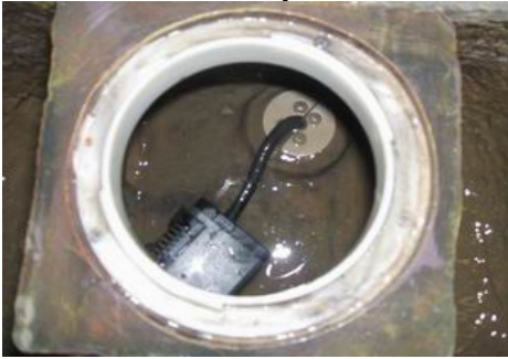
Pump comes pre-installed with cord seal. Check to ensure the cord seal is tight.
