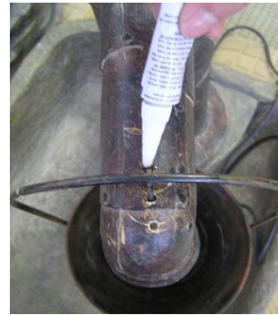
Apply silicone as needed to seal bucket into place.
