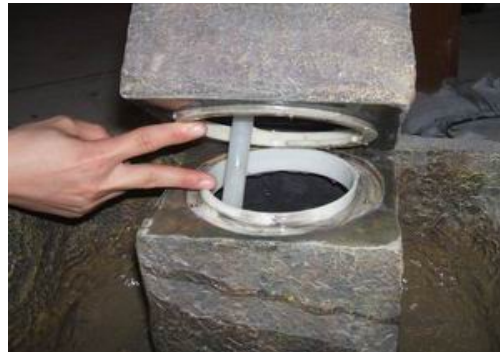
Twist and lock riser to pump house.
