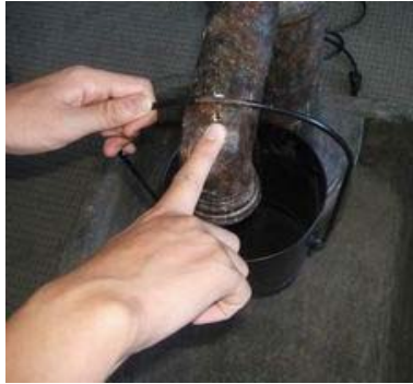
Install spill bucket using grooves. Position bucket so it will spill forward.
