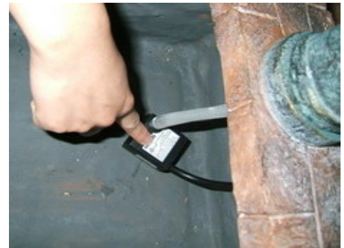
Pump should sit flat and move free inside pump house.
