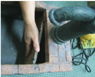
Install the pump access door.
