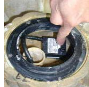
measure amount of tubing needed
