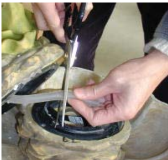
cut tubing to size
