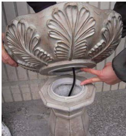
Align and secure the bowl to the pedestal.
