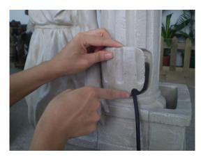
Install the pump access door as shown.
