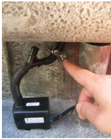
Use the restrictor to the amount of flow from the feature.
