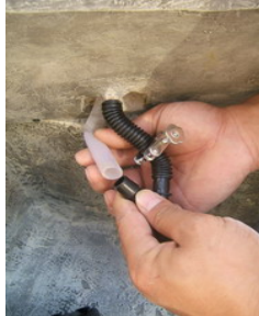
Connect the pre-installed tubing from the "Y" connection to the metal fitting. Connect the tubing from the top to the remaining output of the "Y".
