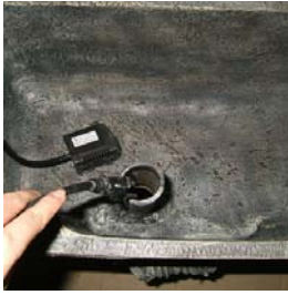
Feed the pump cord down the cord pipe.
