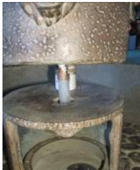
Slide middle riser in place. Pump tubing down to pump.
