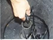
Place the pump inside the reservoir. Feed the light and pump cords down through the cord pipe.
